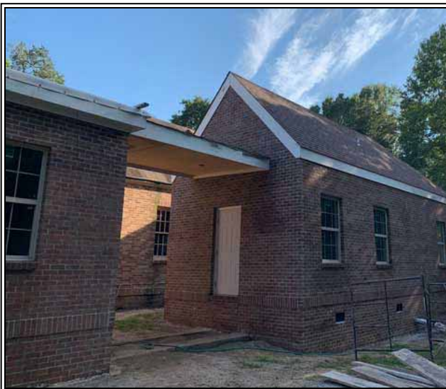
Rear view of the classroom addition
